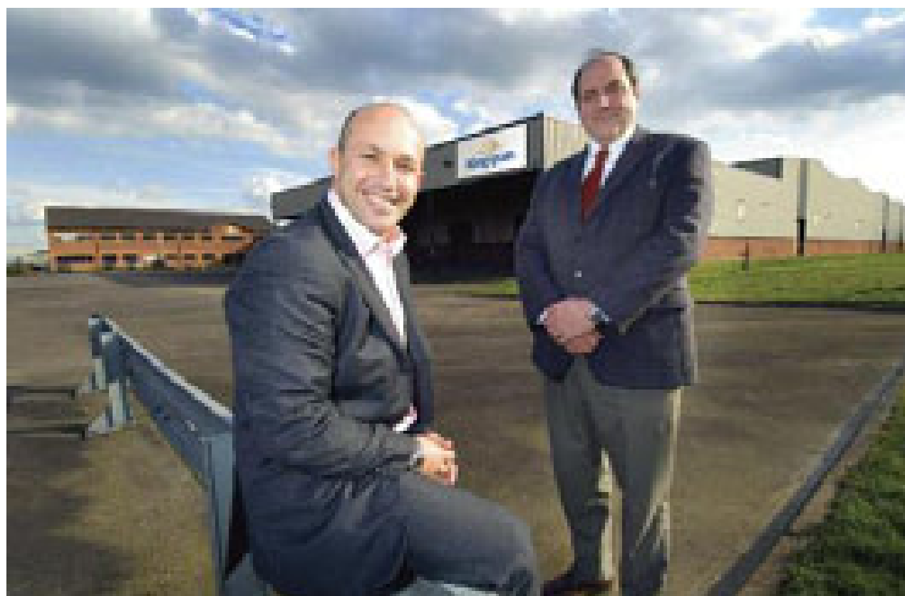
The Selby plant started operation during 2008.
