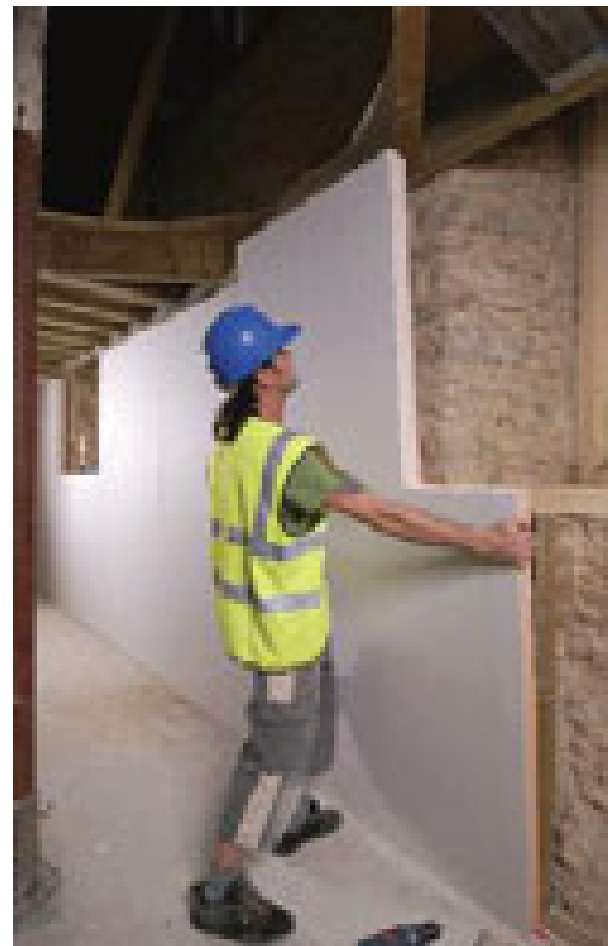
Kingspan Kooltherm K18 Insulated Plasterboard can be used to thermally upgrade solid walled properties. It is mechanically fixed onto a batten framework making it extremely versatile.
