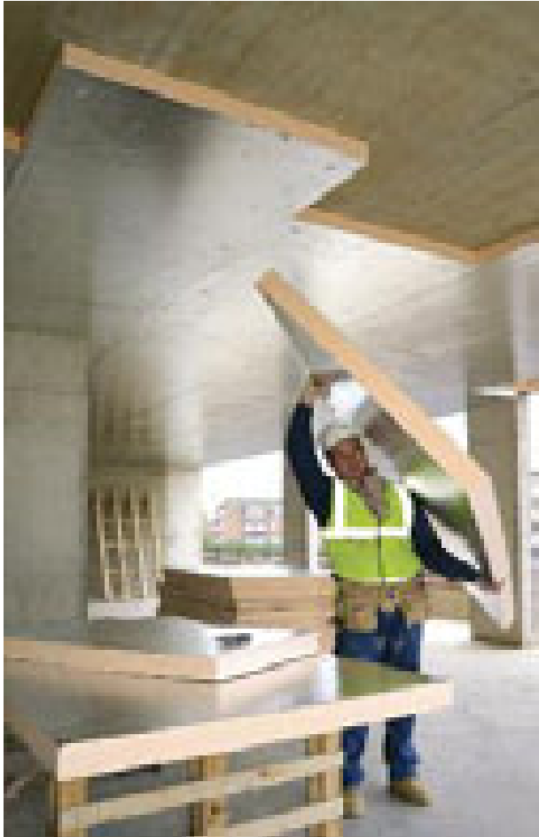
Kingspan Kooltherm K10 Soffit Board is lightweight and easy to install making it the product of choice for soffit applications.
