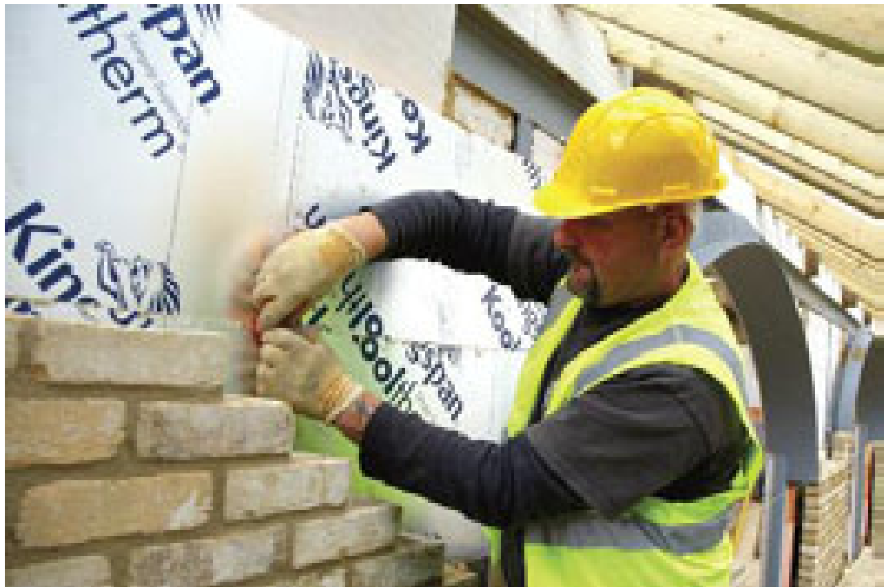
Kingspan Kooltherm K8 Cavity Board is the thinnest commonly used cavity wall insulation material.
